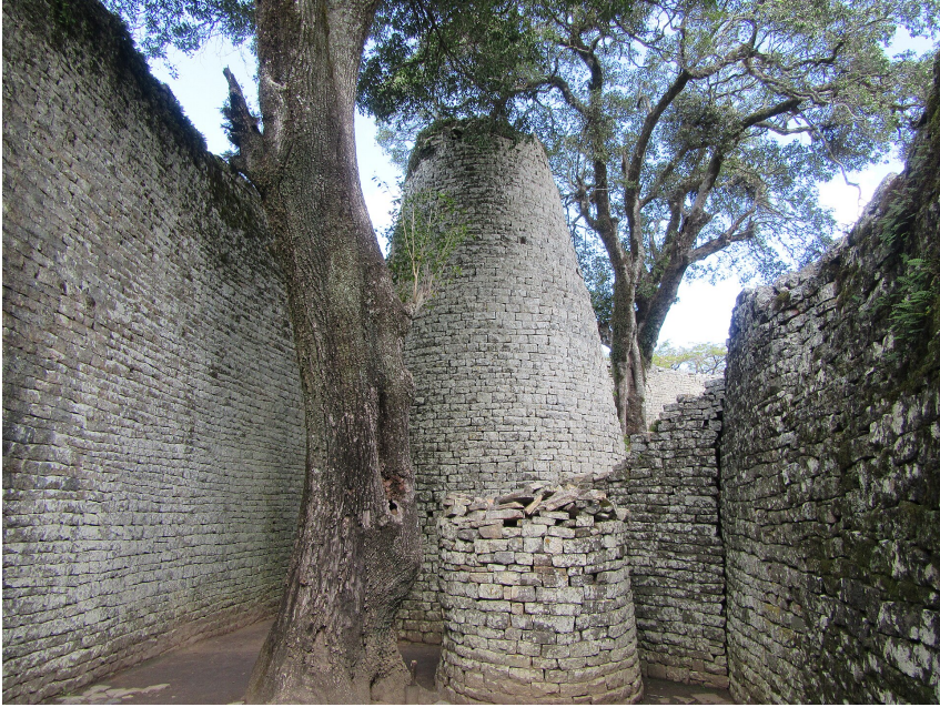
The Conical Tower, Great Zimbabwe – mortarless masonry.
